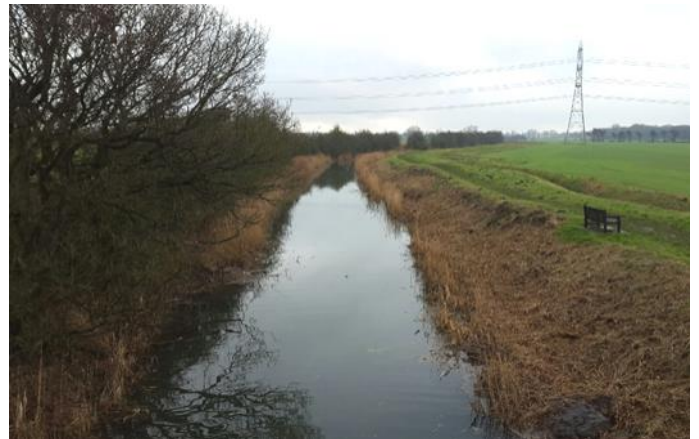
The view from Coates Bridge before (top) and after (bottom).
